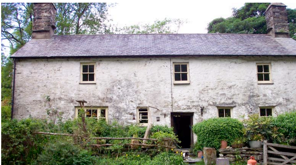
The Hafod Lwyfog farmhouse: a Grade 2* listed building
